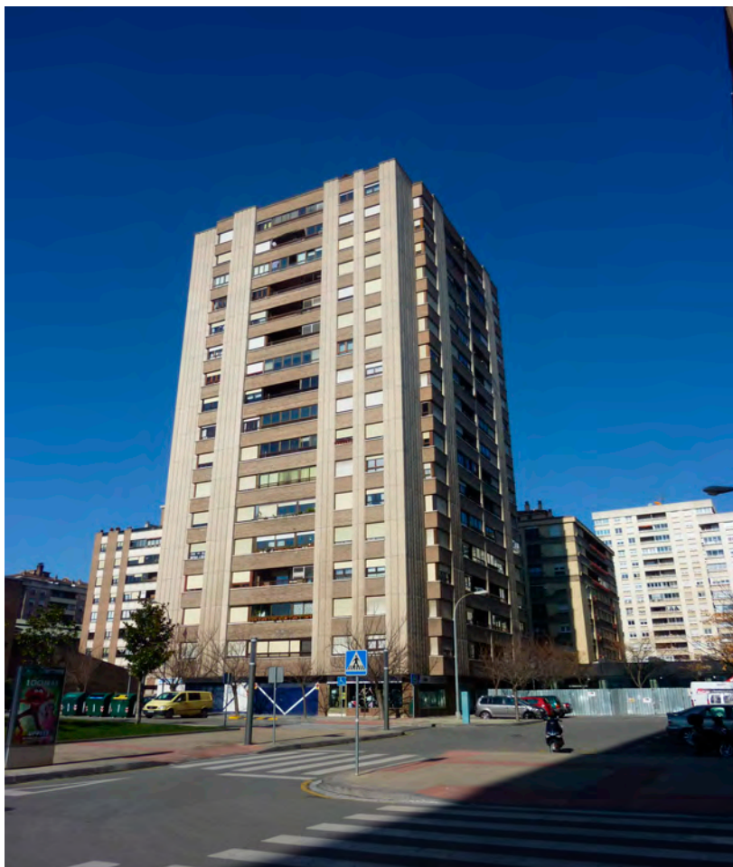
Figure 1. Case study tower's photo.
